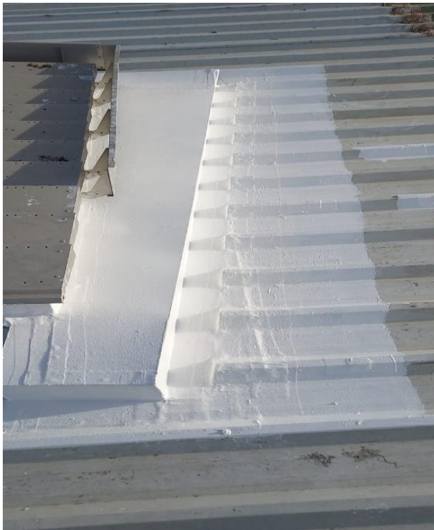
Apply second coat of Thermilate e-coat on complete box
